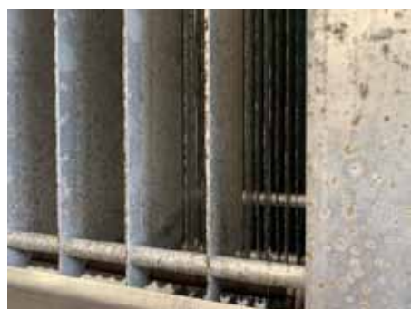
low grade aluminium cell showing signs of rust in a RydAir unit (AOS Australia)
