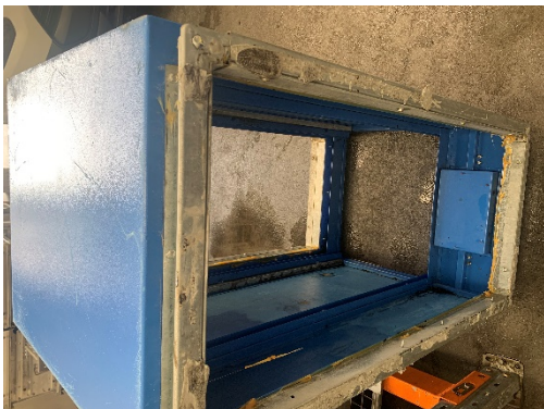
Rydair unit casing (AOS Australia) show no internal slope or internal grease capture capacity meaning the unit increases the build-up of grease in the exhaust system. Unit is made in 1.4mm galvanised steel.
