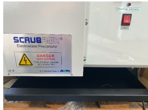
SCRUBBOX unit (AOM Australia) showing the internal grease tray which is located under the unit and out of the exhaust flow. An internal sloping system means that these units extract up to 2-3 litres of grease per day in certain applications. The units are made of 2 mm galvanised steel meaning that they are more durable than the RydAir units.
